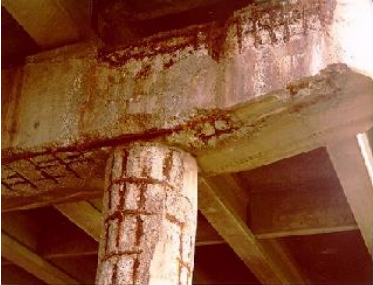
Corrosion
