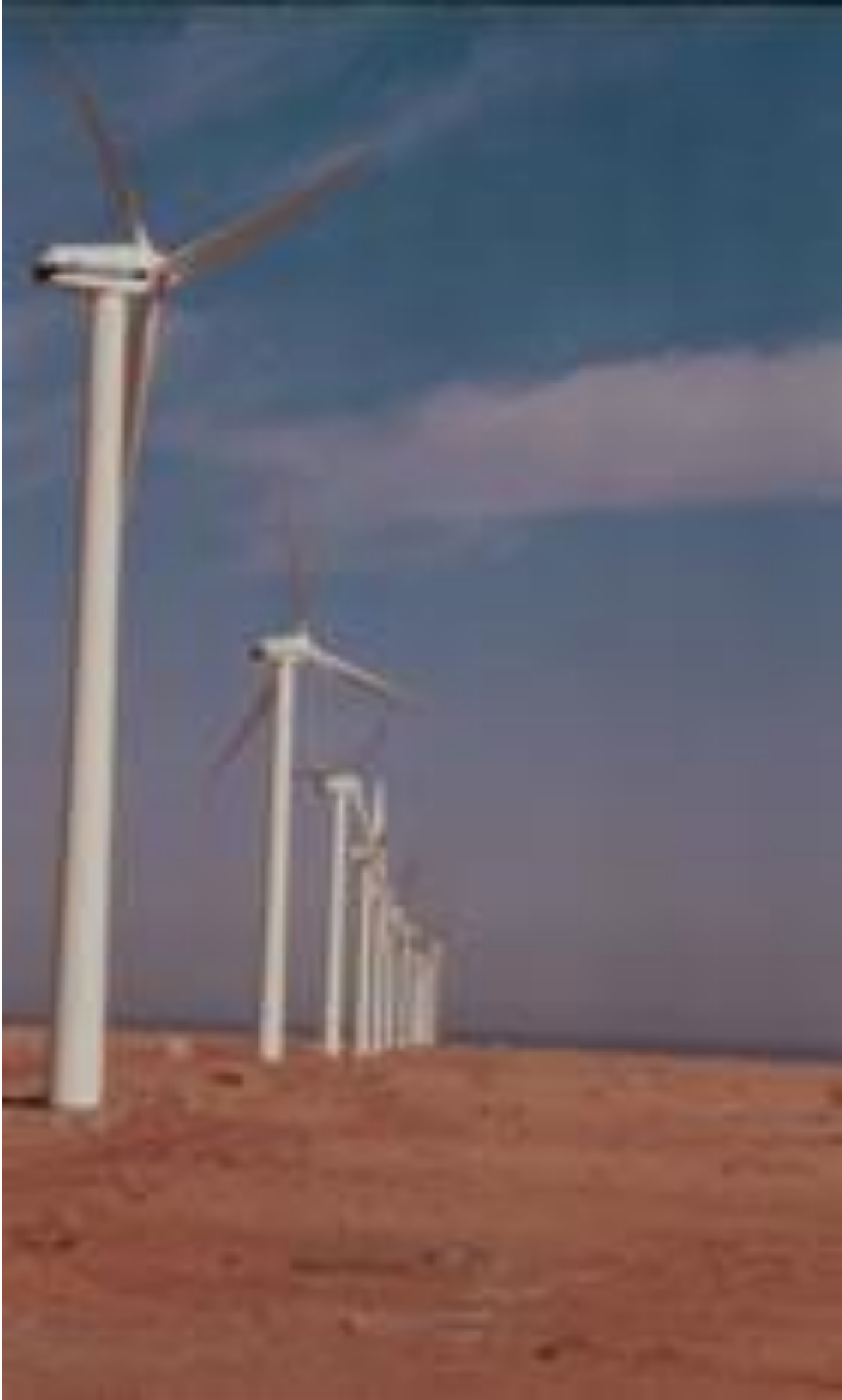
Overview for Zafarana wind farm
