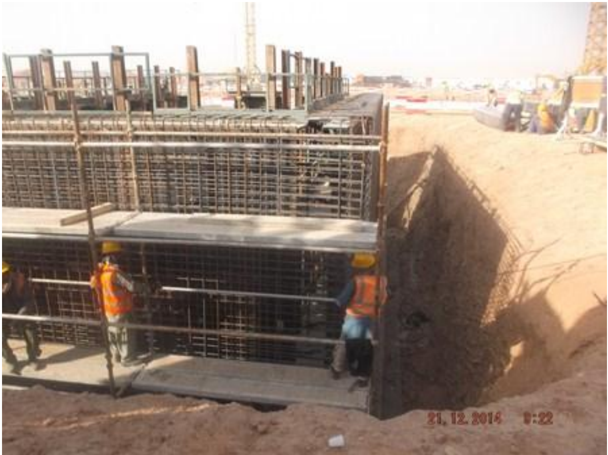
GENERAL VIEW OF TANK
