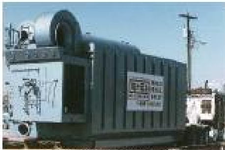
Watertube Boiler D-Type
