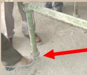
Fig. 4.1 A. Two views of compacted ground or similar soil conditions. Leg located central of mud sill. B. On concrete a base plate is necessary but the mud sill may be omitted.
