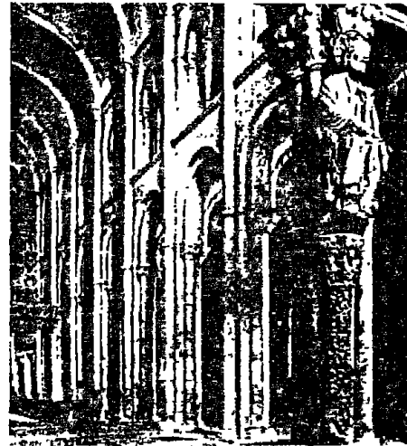
ROMANESQUE. SPAIN. View of the nave, Santiago de Compostela. End of the 11 th century – beginning of the 12 th century.
